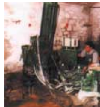
Working from inside the buildings.
