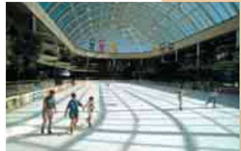
Commercial building, pillars and slabs structure.
