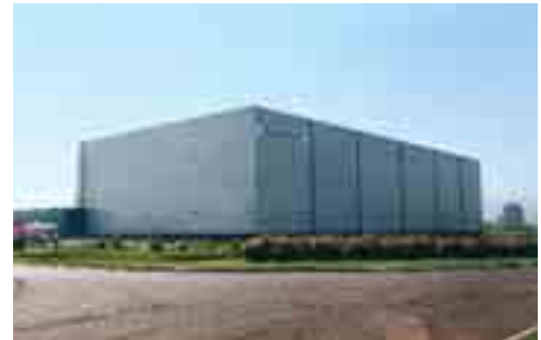
Outside view of a logistic warehouse founded on DR™ pillars.
