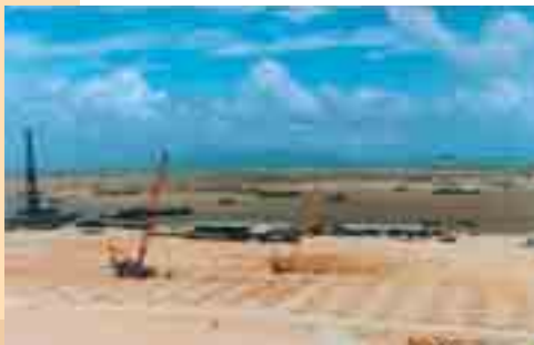
Dynamic Compaction of Macau International Airport's apron.
