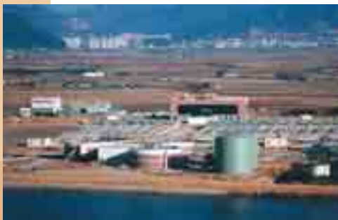
Pusan sewage treatment plant after heavy tanks soil improvement and construction (Korea).
