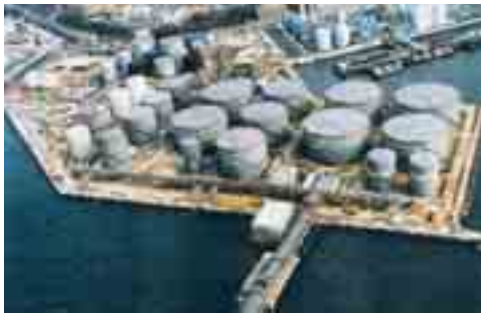
Consolidation using preload & dynamic replacement in Tsing I & II Hong Kong oil storage. (China Petroleum Company)
