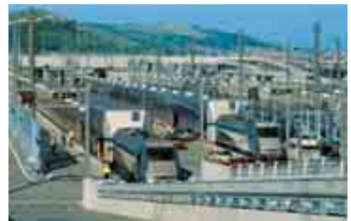
Strengthening by Vacuum™ of the Eurotunnel rail station at Coquelles (France). View of the station after construction.
