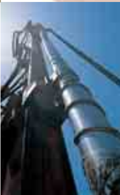
Controlled Modulus Columns
