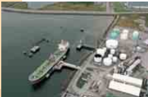
Turnkey foundation system including preloading, Dynamic replacement under infrastructures. Jet grouting under heavy tanks.
