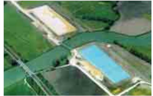
Menard Vacuum consolidation™ under the Boutonne river of approach embankments for A537 expressway (France).
